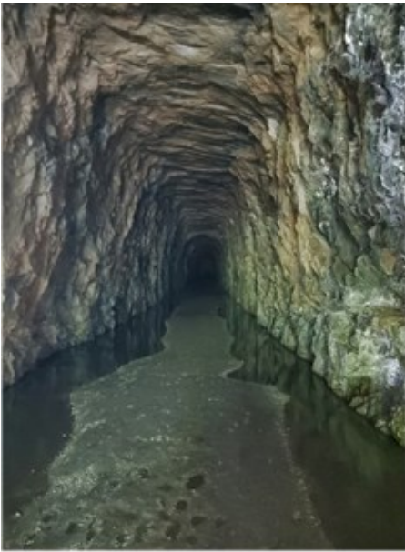
SC Blue Ridge Railroad's Unfinished Stumphouse Mountain Tunnel, July 2020
