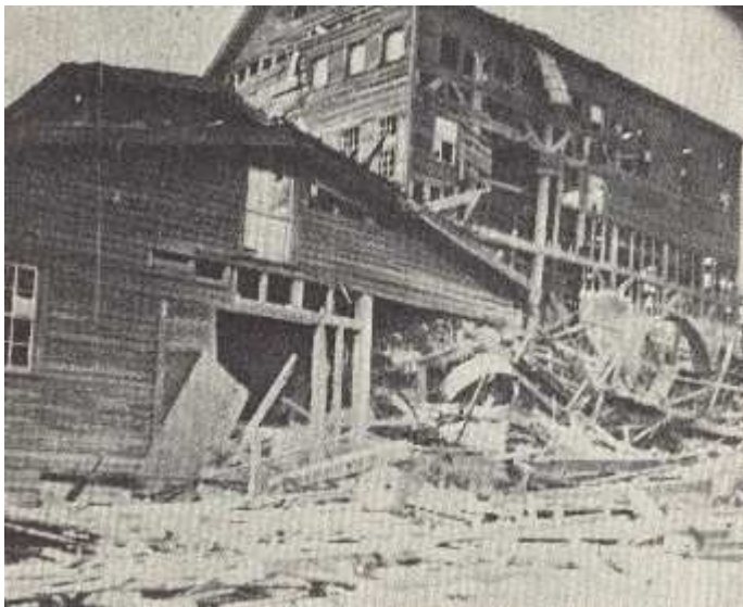
Southeast view of the stamp mill plant made a few days after the boiler explosion - August 1908.
